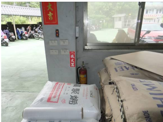
A fire extinguisher is blocked by pallets of goods.
